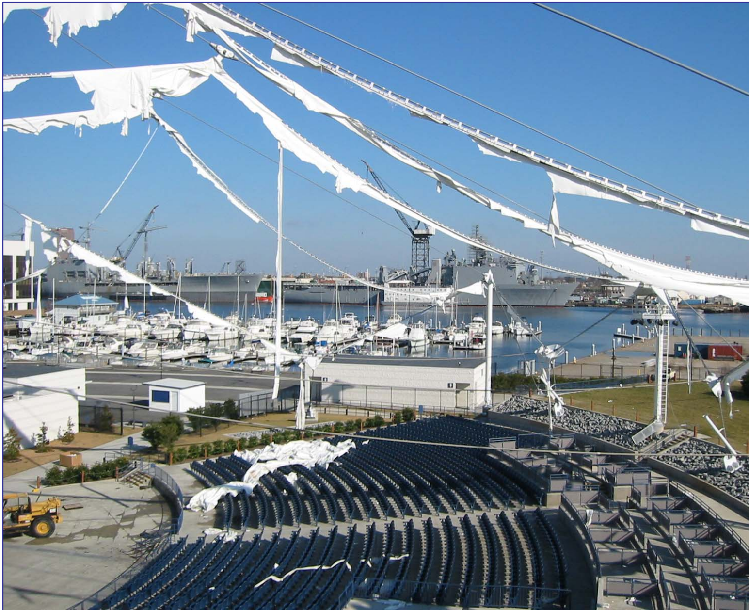
Open air theatre destroyed by a hurricane (Portsmouth, Virginia, USA)
